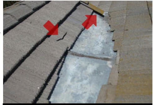
Rake tile blocking valley water runoff.
