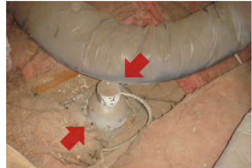
3" of seperation is required if Non IC.
