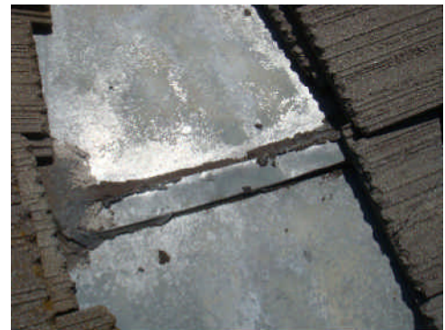
Tile blocking water runoff.
