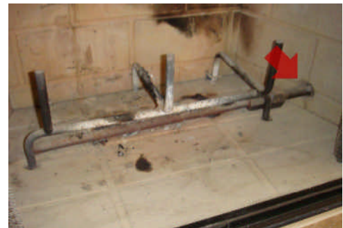
Seal around the gas pipe.
