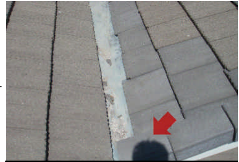
Tile blocking water runoff.
