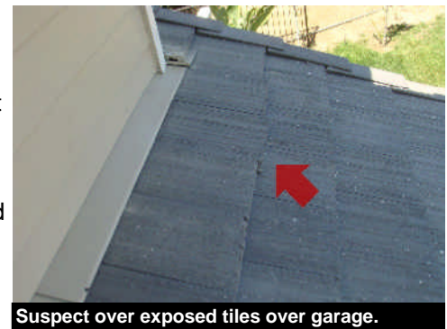
Debris over the garage & broken tile edge.
